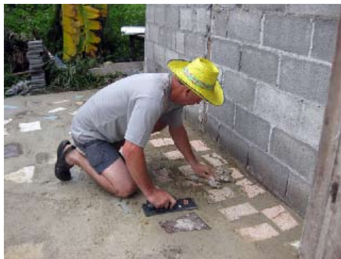
Brian starts work on a slum dwelling
